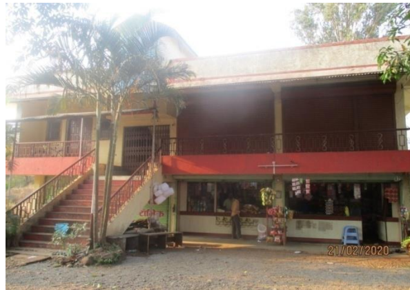
Figure 5.28 Front view of the two-storey RC building
