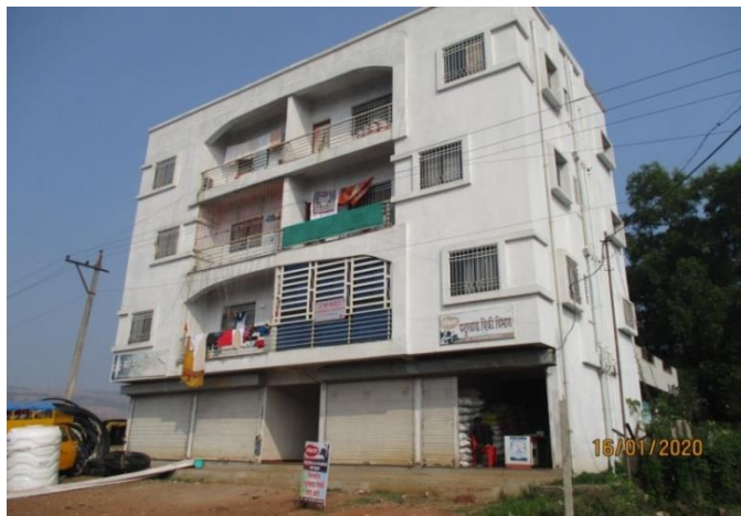
Figure 5.10 Front view of the four-storey RC building
