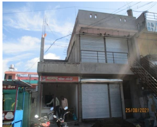
Figure 5.25 Front view of the three-storey RC building
