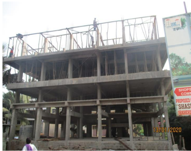
Figure 5.49 Front view of the four-storey RC building
