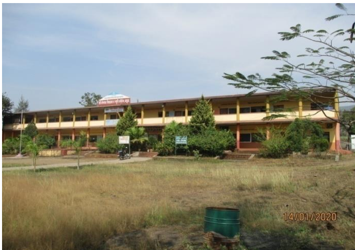
Figure 5.43 Front view of the two-storey RC building
