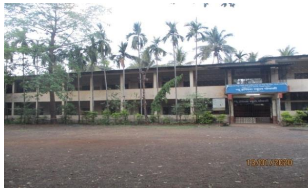
Figure 5.52 Front view of the two-storey RC building
