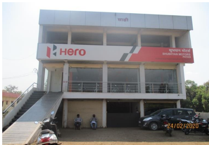
Figure 5.16 Front view of the three-storey RC building
