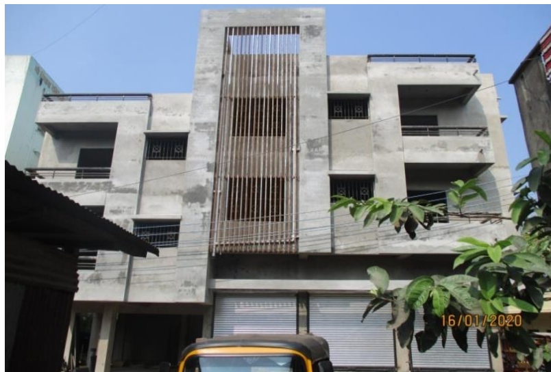
Figure 5.2 Front view of the three-storey RC building
