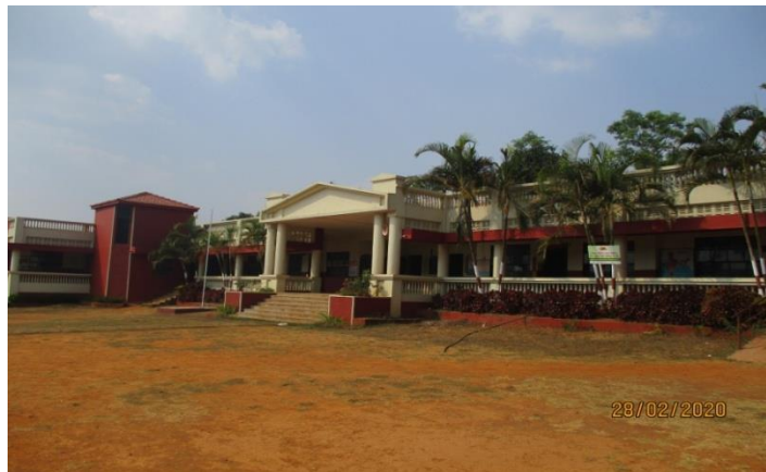
Figure 5.13 Front view of the single-storey RC building
