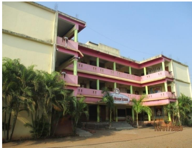
Figure 5.40 Front view of the three-storey RC building
