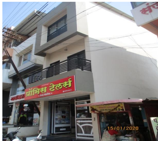
Figure 5.19 Front view of the three-storey RC building
