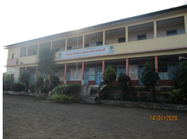
Figure 5.46 Front view of the two-storey RC building
