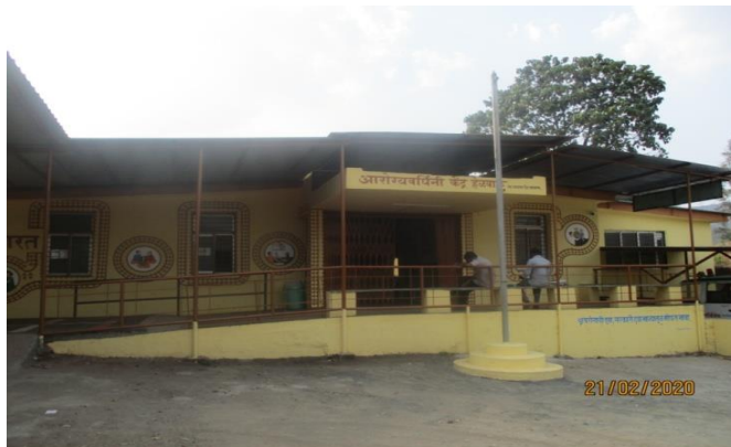
Figure 5.37 Front view of the single-storey RC building
