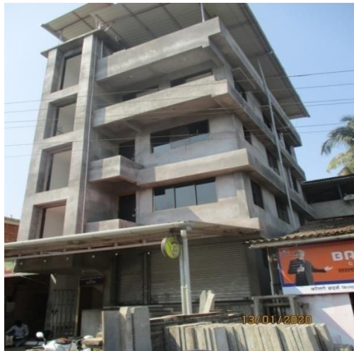
Figure 5.22 Front view of the five-storey RC building
