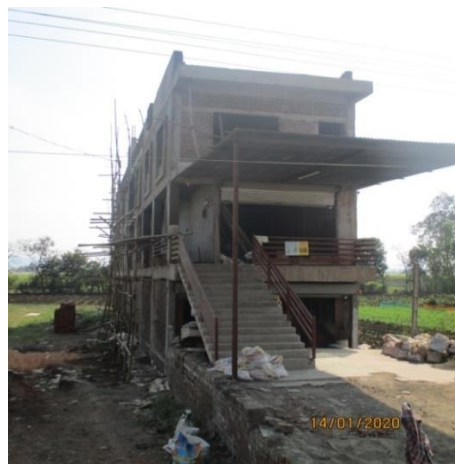
Figure 5.34 Front view of the three-storey RC building
