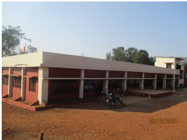
Figure 5.31 Front view of the single-storey RC building
