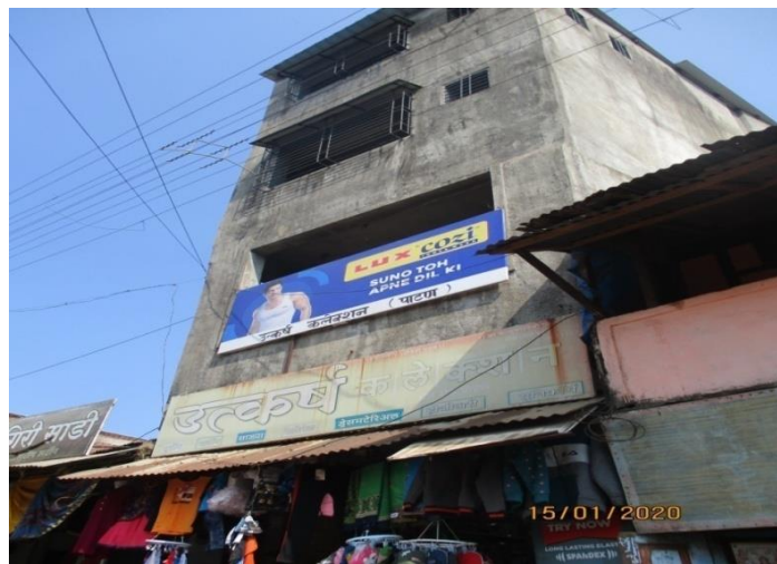
Figure 5.7 Front view of the four-storey RC building
