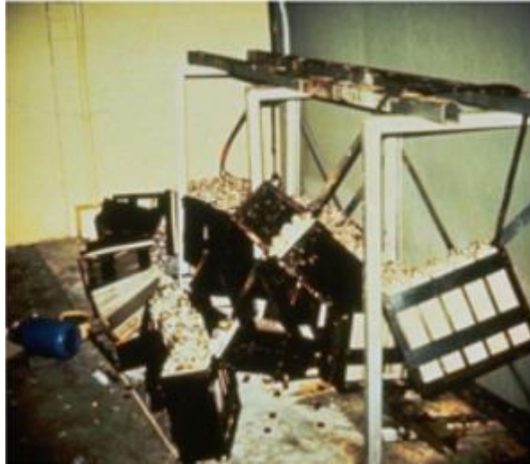
Figure 1.7 Poor earthquake performance of NSEs 1971 San Fernando Earthquake [12]
