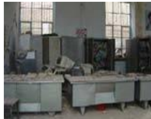
Bam 2003 (Bam Earthquake Report 2003)
