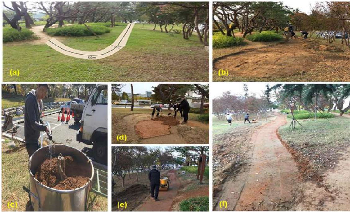
Figure 4.4 Overall procedure of earth stabilization using biopolymer solution (Daejeon, Korea; October 2015)
