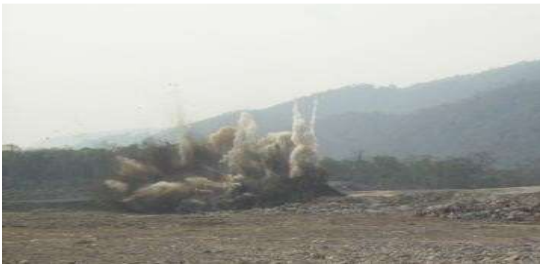
Figure 3.12: Blasting operation in Quarry 'B'
