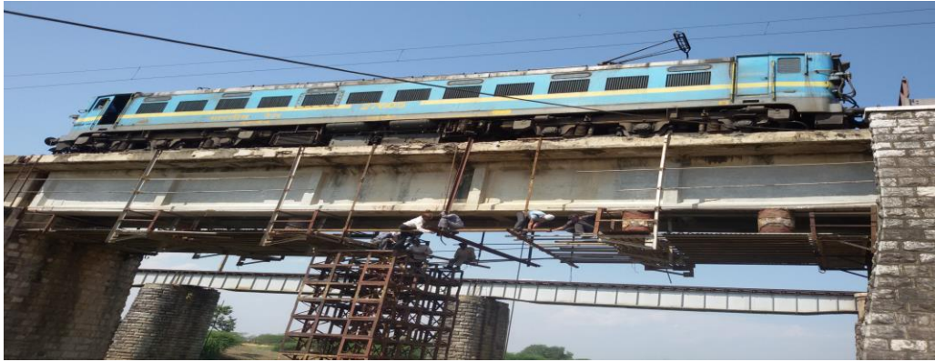
Figure 5. 57 Load applied on the bridge using wagon 7 and sensors at site
