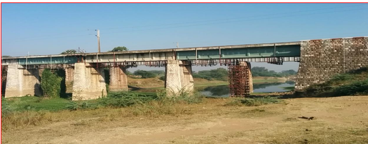
Figure 5. 1 Site view of bridge no 114
