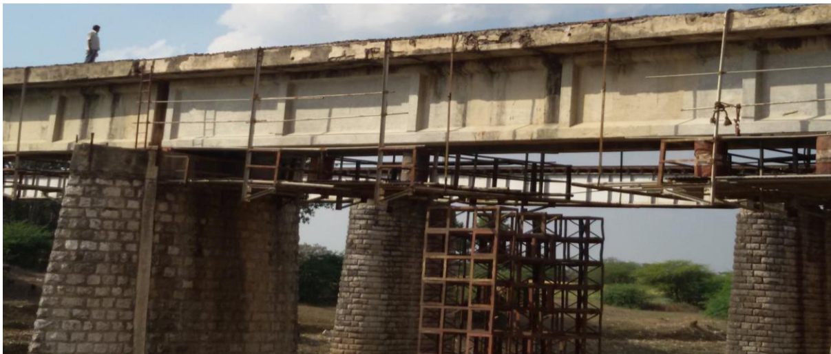
Figure 5. 50 View of bridge no 54 at site
