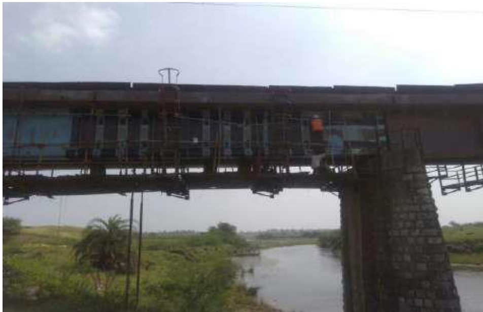
Figure 5. 37 strengthening using fibre at site of bridge no 114
