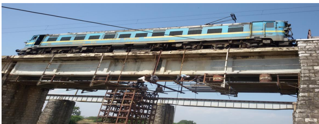
Figure 5. 38 Load applied on the bridge using wagon 7
