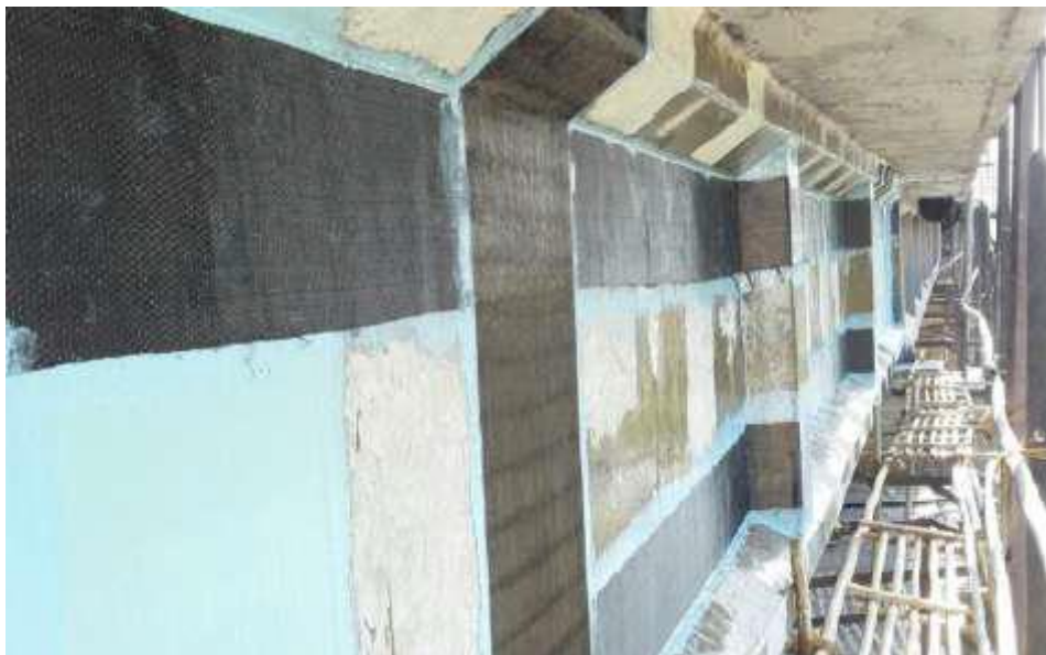
Figure 5. 56 Lamination of bridge no 54 at site
