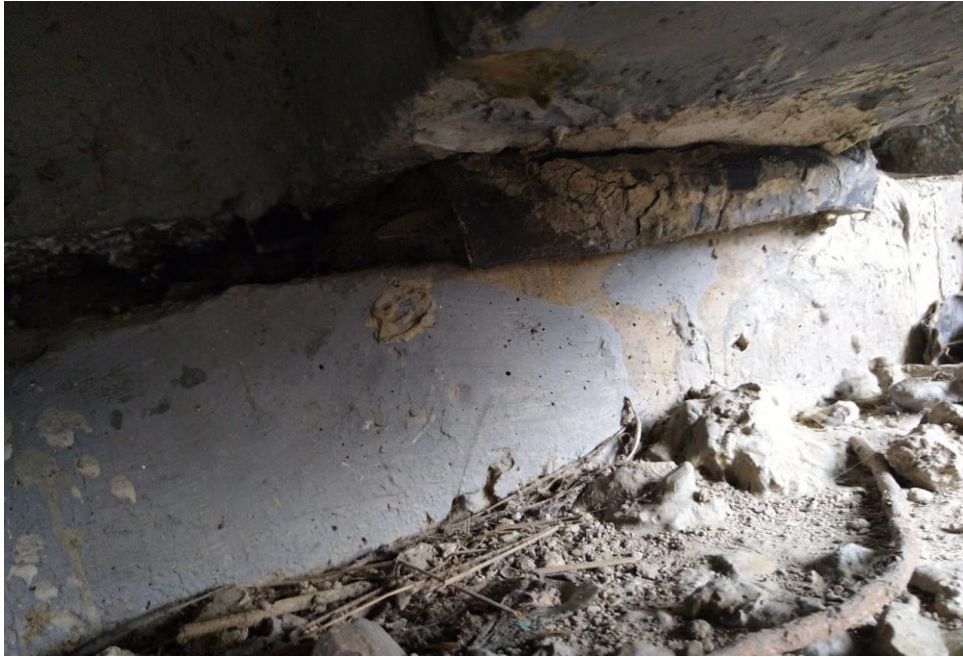
Figure 4. 6 Stifling of bearing
