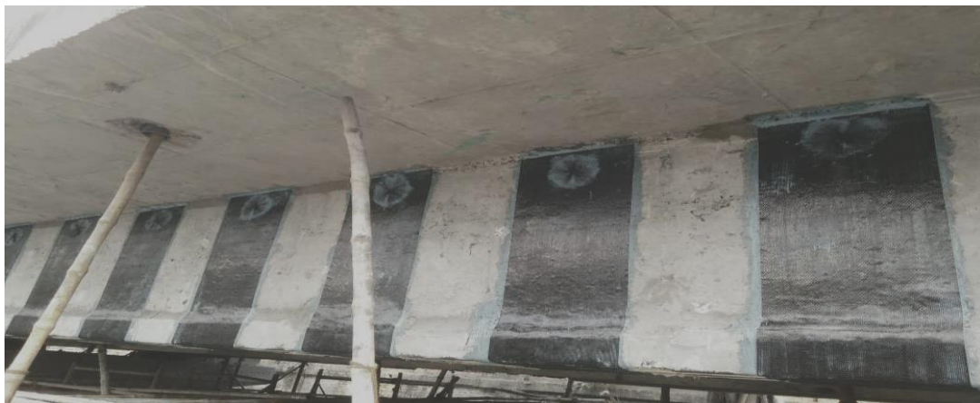
Figure 4. 40 Treatment of exposed reinforcement and Anti-corrosive paint
