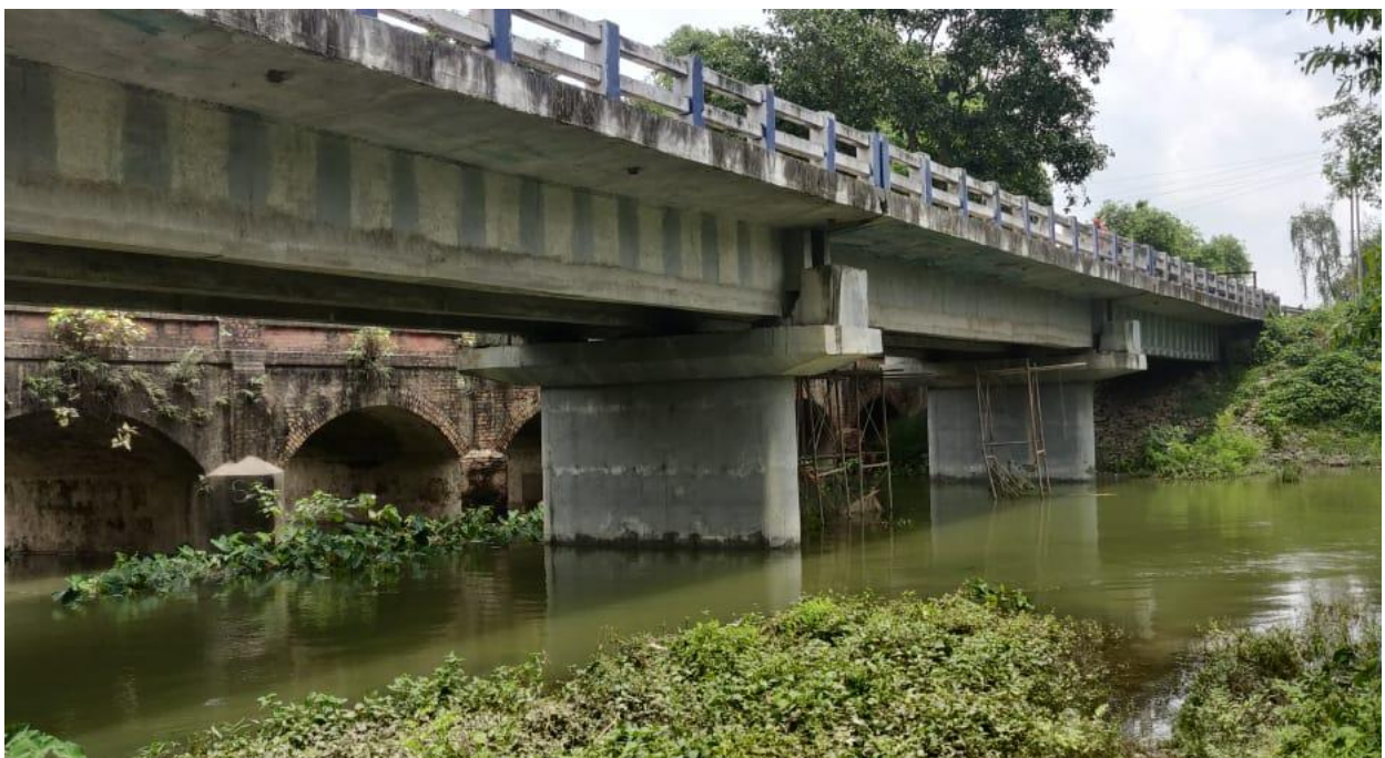
Figure 4. 1 View of Pusa-Muzaffarpur bridge
