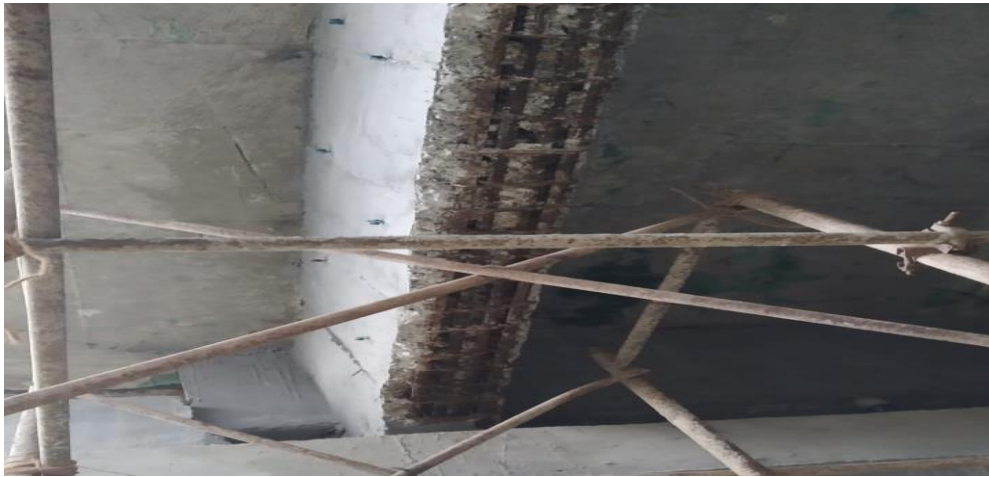
Figure 4. 39 Side view of strengthening scheme of Girder
