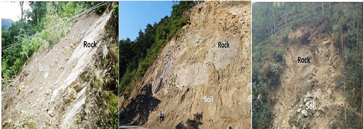
Fig. 3.6. Failure of the entire residual soil layer observed at various sites in the study area
