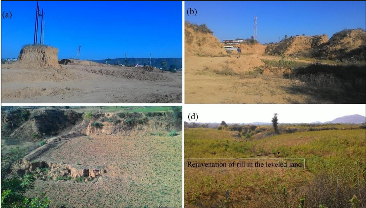
Figure 7. 12 Field photographs showing (a) and (b) Levelling of land by cut and fill method; (c)and (d) Rejuvenation of rills and gully in freshly reclaimed land by cut and fill method
