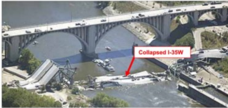
Figure 2.7 Failed superstructure of I-35W bridge [A. Astaneh-Asl, 2008]
