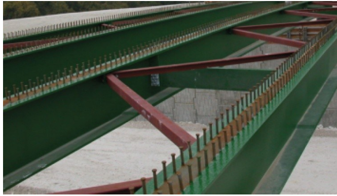
Figure 2.29 Headed shear connectors
