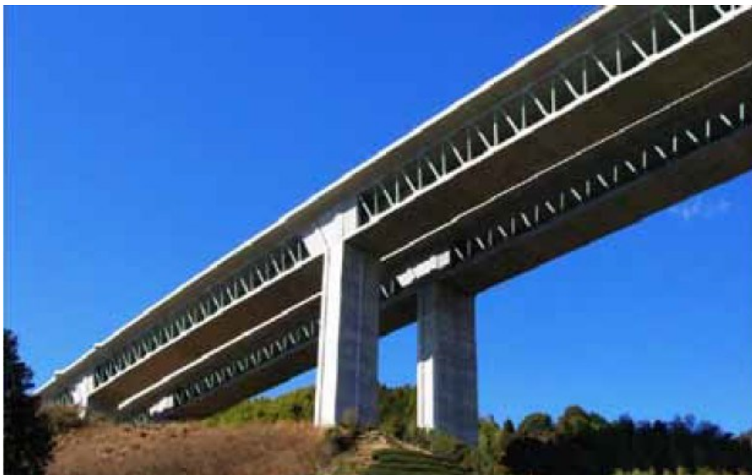
Figure 2.24 Sarutagawa bridge [K. Ohgaki, 2011]
