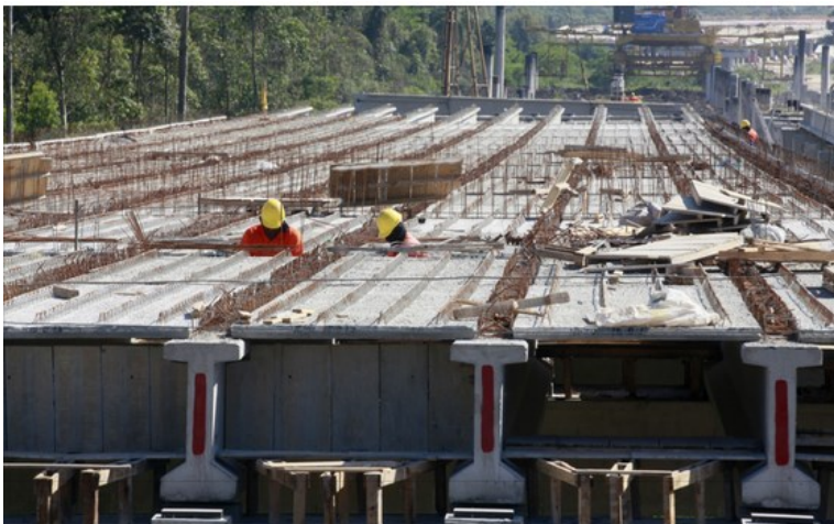
Figure 2.28 Anchorage shear connectors
