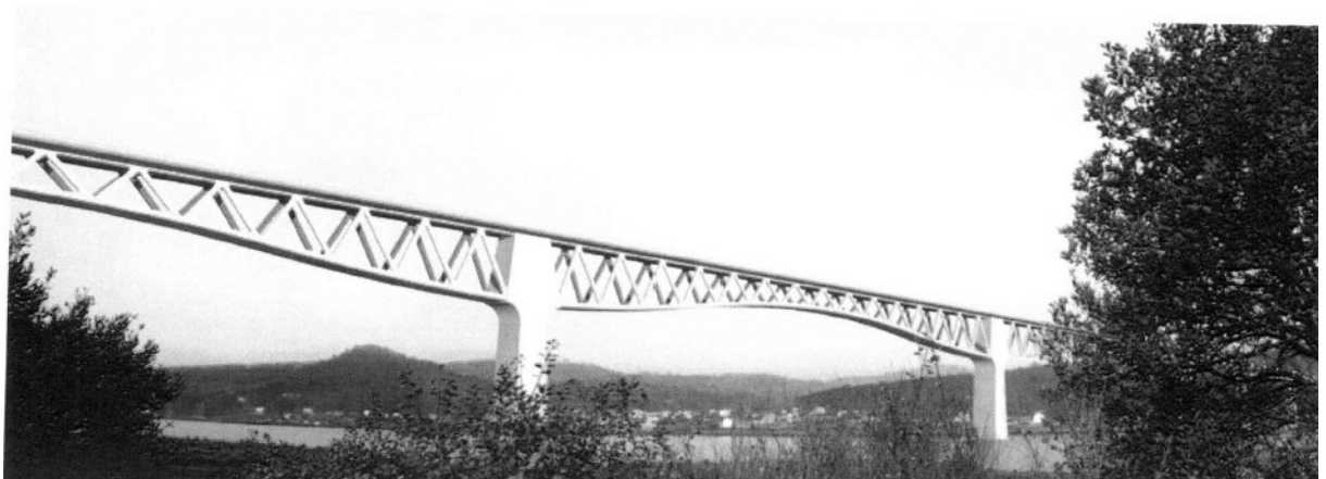
Figure 2.23 View of the Ulla river viaduct [F. Millanes, 2010]
