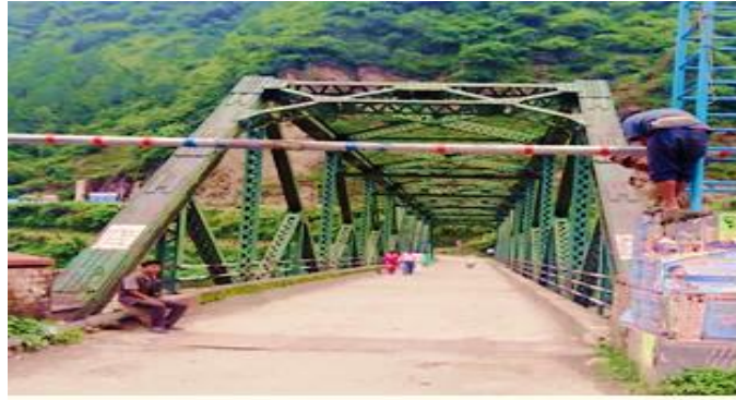
Figure 3.1 Picture of the selected steel truss bridge situated in Uttarkashi, India
