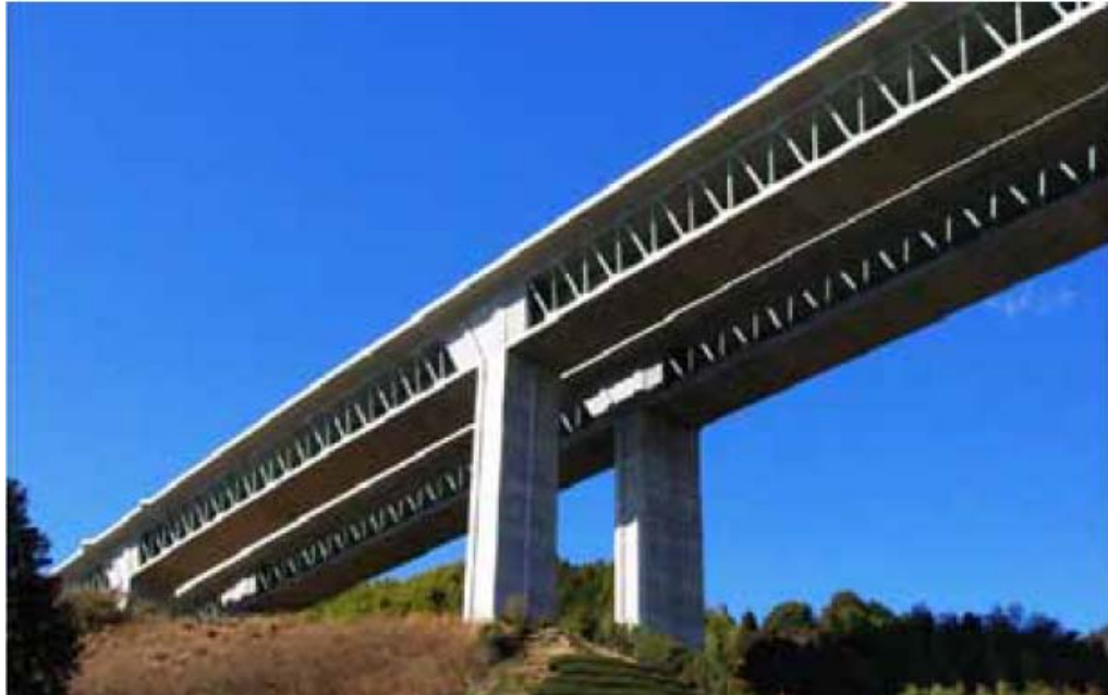
Figure 2.8 Sarutagawa Bridge (K. Ohgaki, 2011)
