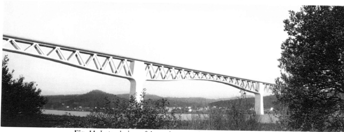
Figure 2.7 View of the Ulla river viaduct (F. Millanes, 2010)
