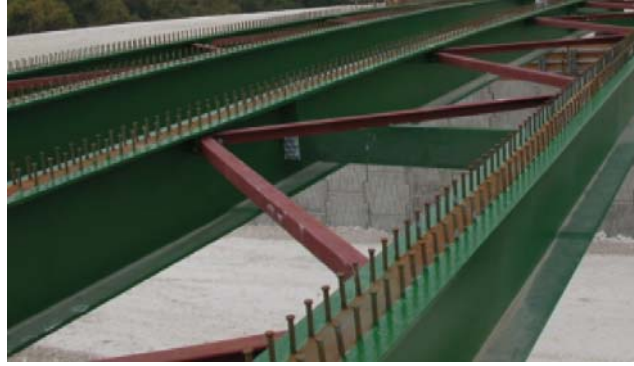
Figure 2.13 Headed shear connectors (A41 Aston Clinton Bypass)
