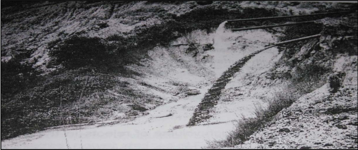
Fig. 2.2: Disposal of Flyash slurry through pipe line from TTPS into residual quarry of Balanda OCM, MCL
