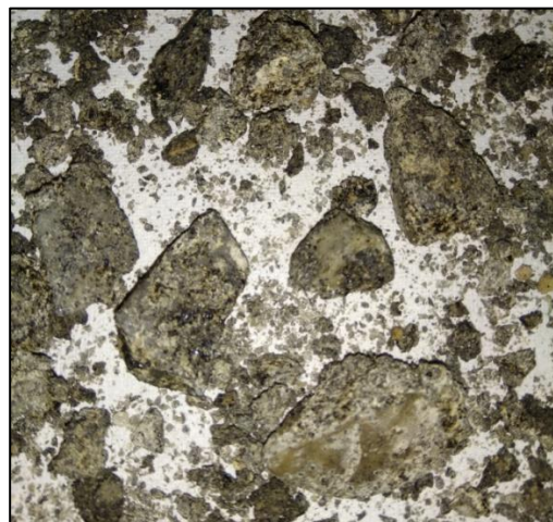
Plate 7.5 Analysis of stripping by visual inspection
