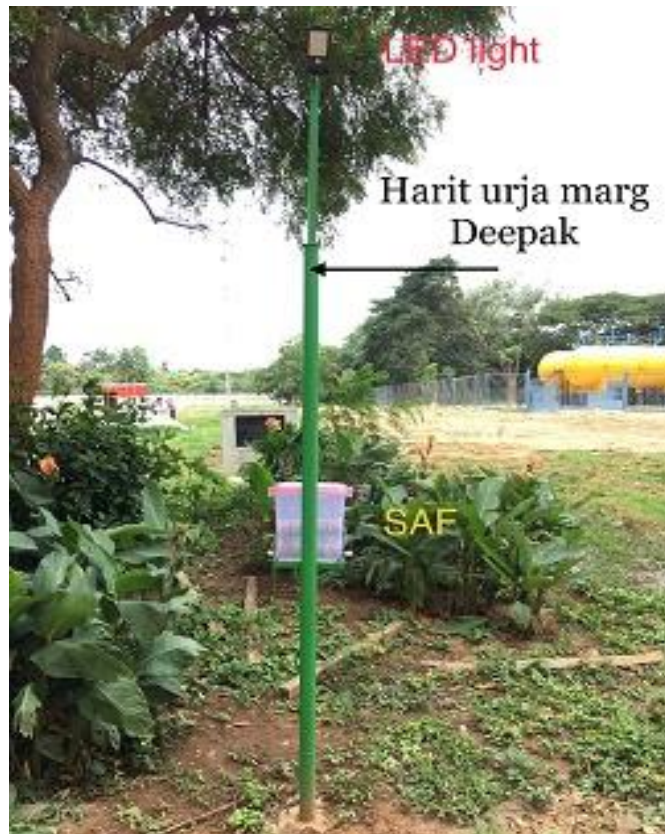
Figure 5.7: Hybrid Bio-Solar Street Light System
