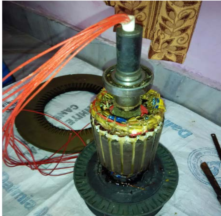
Fig. 3.18 The winding of inner stator coming through the shaft of the generator
